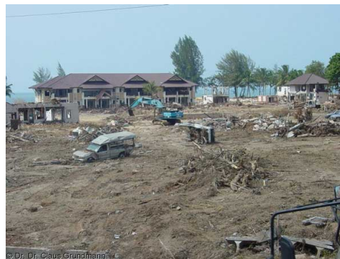
Fig. 9: Destruction by Tsunami
