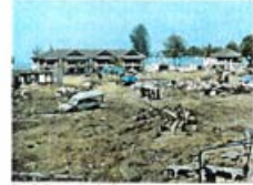
Fig. 9 Destruction by Tsunami
